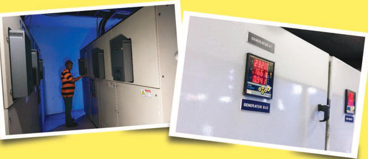
• Power Factor Correction Equipment. •
